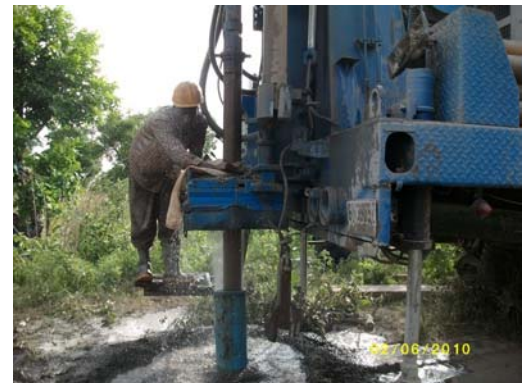
Testing the flow rate of the new borehole in Nyobido—30 liters per minute!
